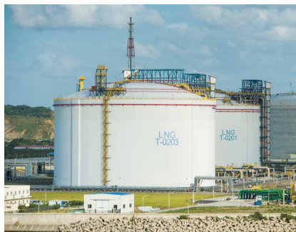
Liquid level tank
